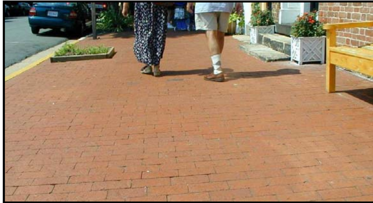
Properly installed and well maintained brick can work.
