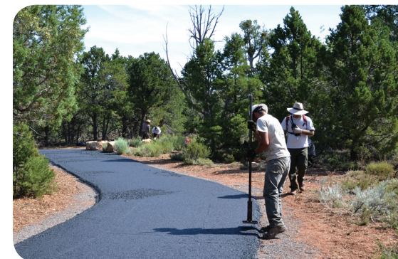
Trail development photo from Grand Canyon National Park Service http://www.flickr.com/photos/grand_canyon_nps/
