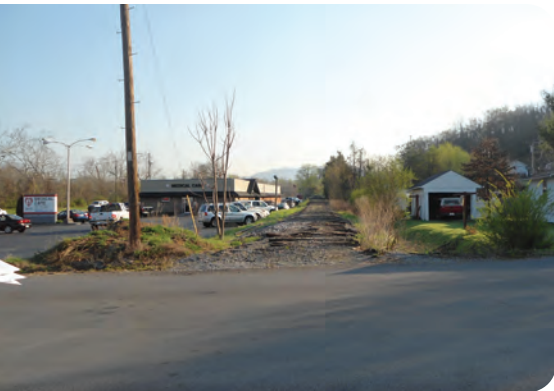
Rail trail crossing at Ward Street, Elizabethton, Tennessee
