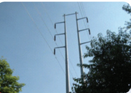
Utility crossings exist along the Johnson City Rail Trail Corridor
