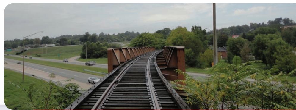
Rail Trail Overpass, over Hwy 67 in Johnson City, Tennessee
