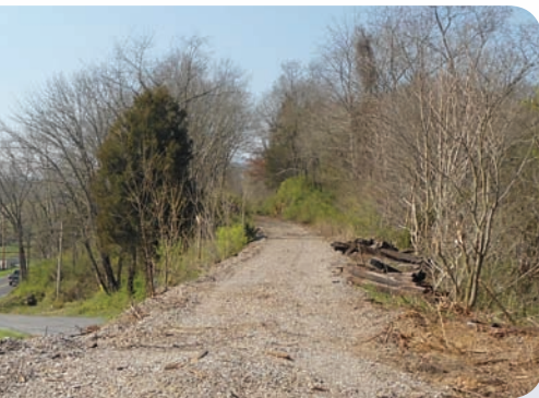
Existing ballast on rail bed, near Happy Valley Road
