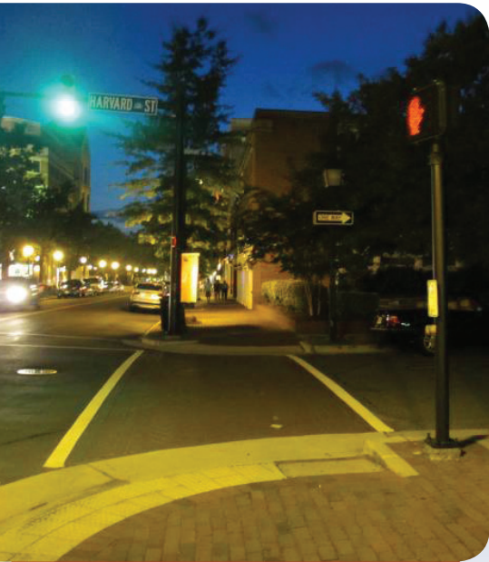
The illumination shown along the street above is not uniform, producing light and dark pockets along the sidewalk. The low pressure sodium lamps cast a yellow light that results in poor color rendition.
