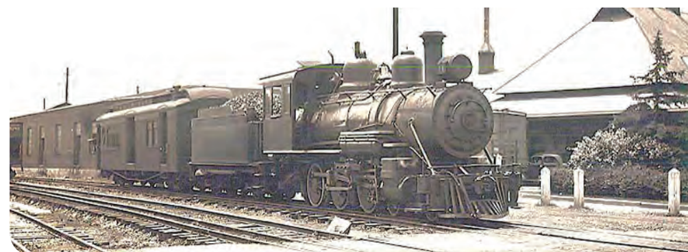
The daily train in Johnson City circa 1930. (Photo from: http://www.johnsonsddepot.com/crumley/tour4.htm )
