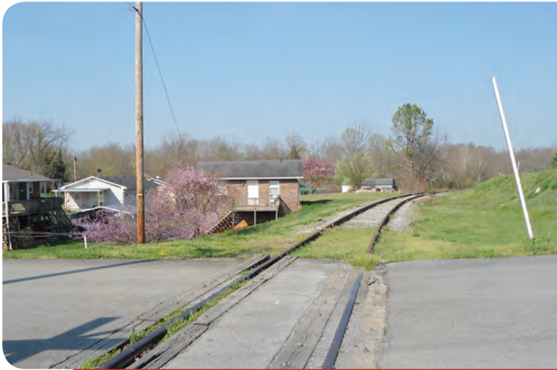
At-grade crossing at Emmanuel Street, Carter County, Tennessee
