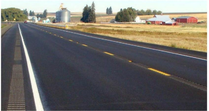
Figure 21: Edge and centerline rumble strips (Source: FHWA)
