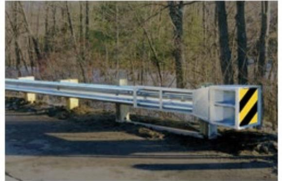
Figure 35: Energy-absorbing end treatment (Source: FHWA, W-Beam Guardrail Repair)
