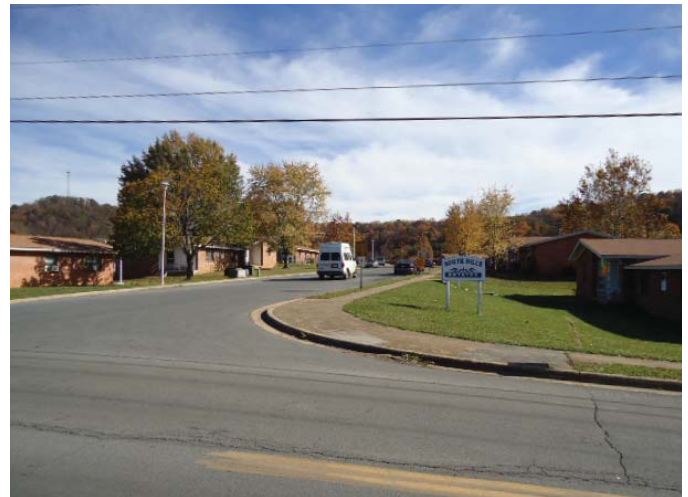
Most higher-density housing is located south of downtown. Multi-family units are not common, though several are either planned or under construction.
