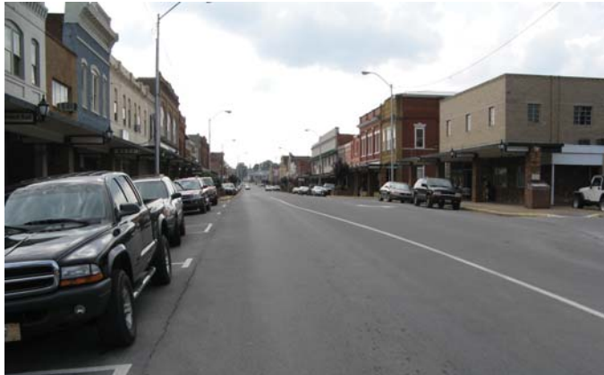
Project M-2. Elizabethton's Downtown Enhancement Plan provides guidance on returning Elk Avenue to two-way traffic. Bike lanes should also be considered downtown. A downtown circulation study would validate the Enhancement Plan findings with technical analysis.
