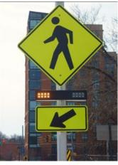
Figure 24: Rectangular Rapid Flashing Beacon (Source: FHWA MUTCD)
